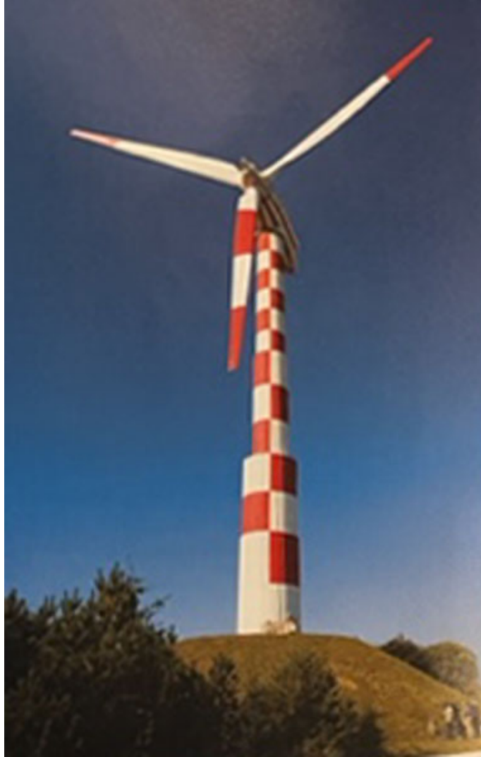
The megawatt wind turbine produced by Twindkraft of the Tvind School on Jutland, Denmark. From Paul Gipe Wind Energy for the Rest of Us . 2016 wind-works.org. p58-68.
